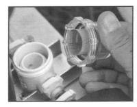
4. Unscrew the cap on the in-line strainer and manually fill it with water to get it started.
